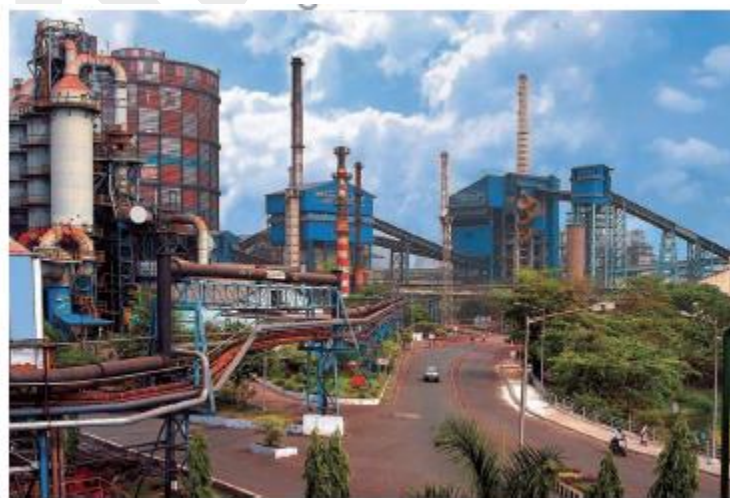
Tata Iron and Steel Company
