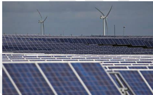
Kamuthi solar power plant
