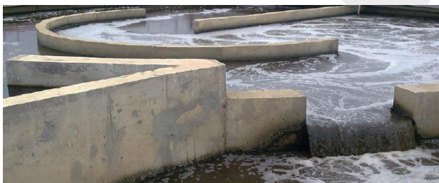
Waste water treatment plant
